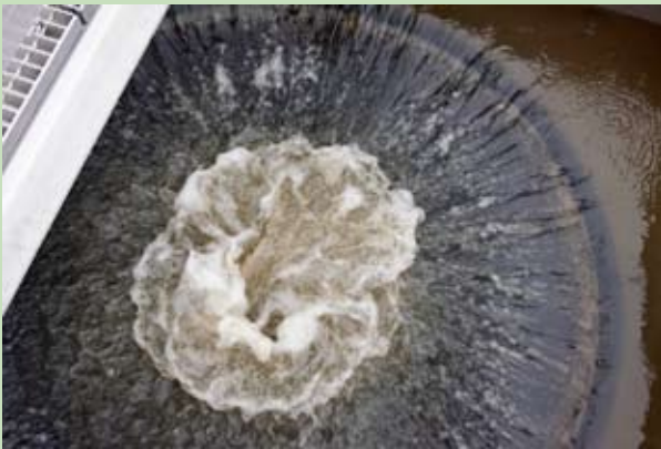
The Storm King®, an advanced vortex separation chamber with a self-cleansing screening system, is designed for use in municipal combined sewer overflows. Locally, this Hydro International product is in operation at the Saco Wastewater Treatment Facility located along the Saco River. Chief Operator John Hart checks the system during a heavy rain event.
