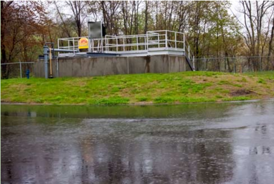
The Storm King®, an advanced vortex separation chamber with a self-cleansing screening system, is designed for use in municipal combined sewer overflows. Locally, this Hydro International product is in operation at the Saco Wastewater Treatment Facility located along the Saco River. Chief Operator John Hart checks the system during a heavy rain event.
